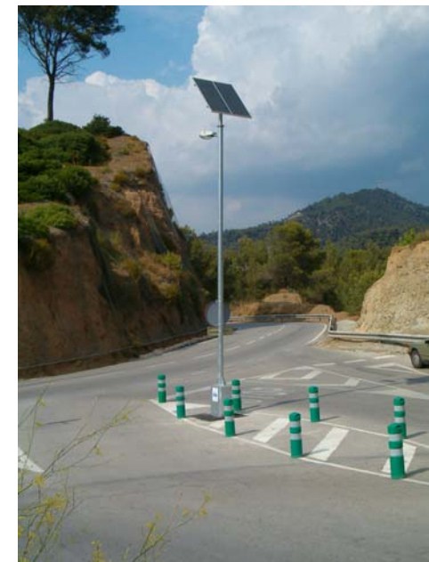
NORDEX Hot galvanized Steam of sodium
